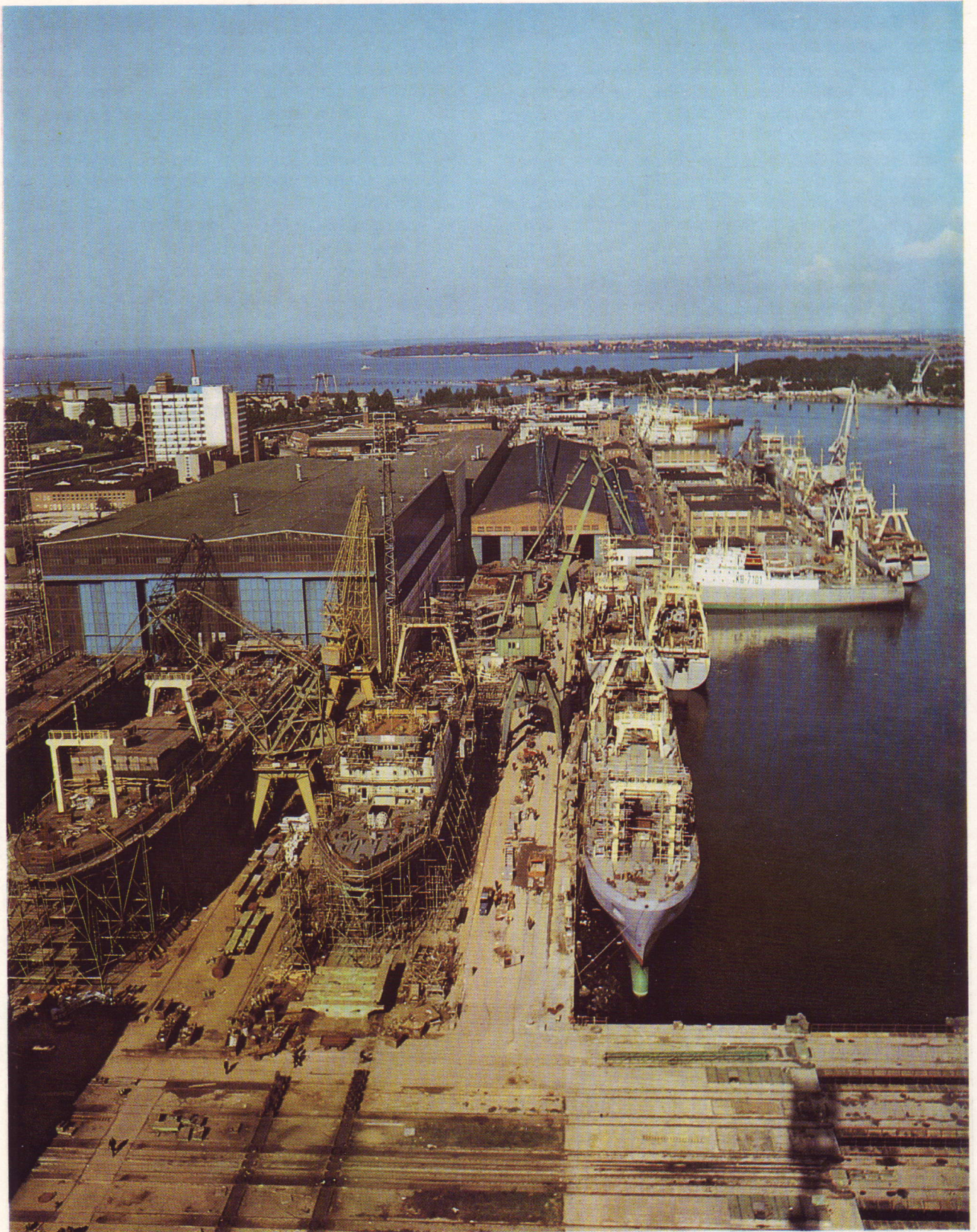
View of the shipyard and of ships being under construction
